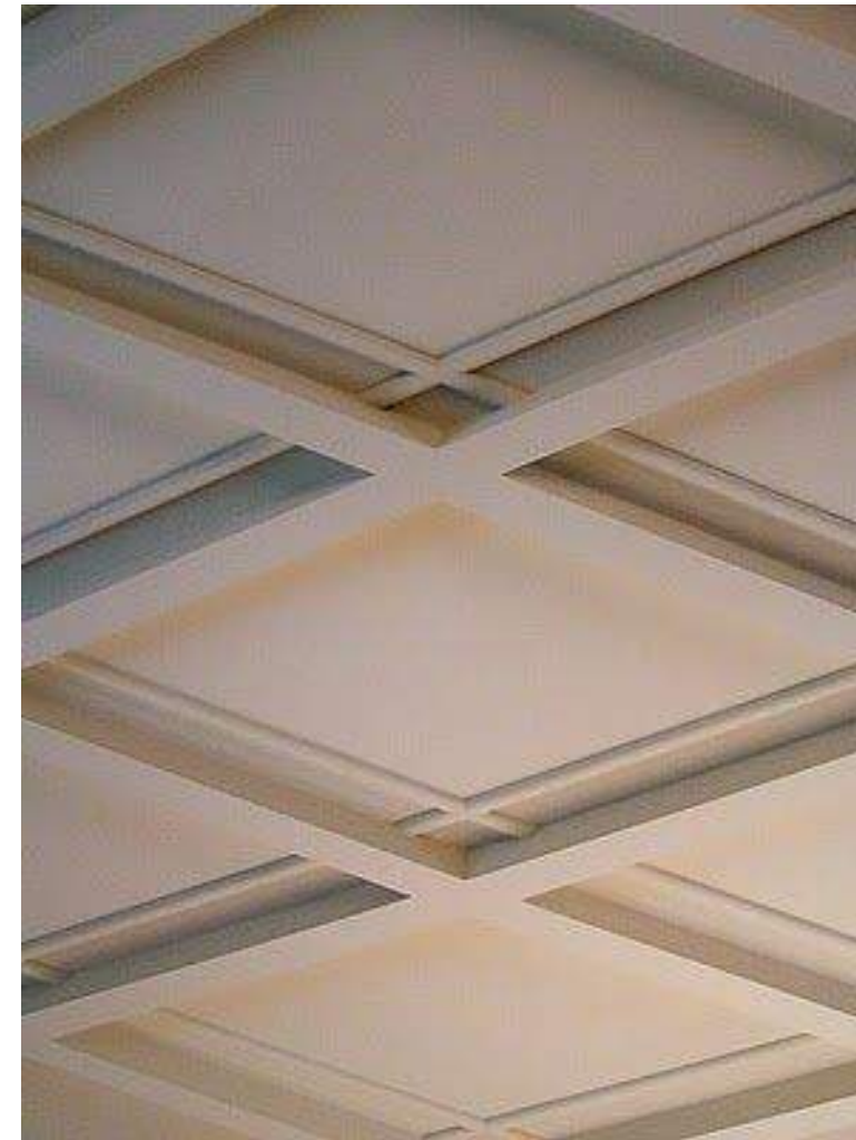
Millwork Panel Ceiling Concept
